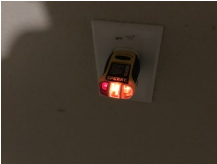
All lights on plug tester lit up and GFCI would not trip in garage outlet
