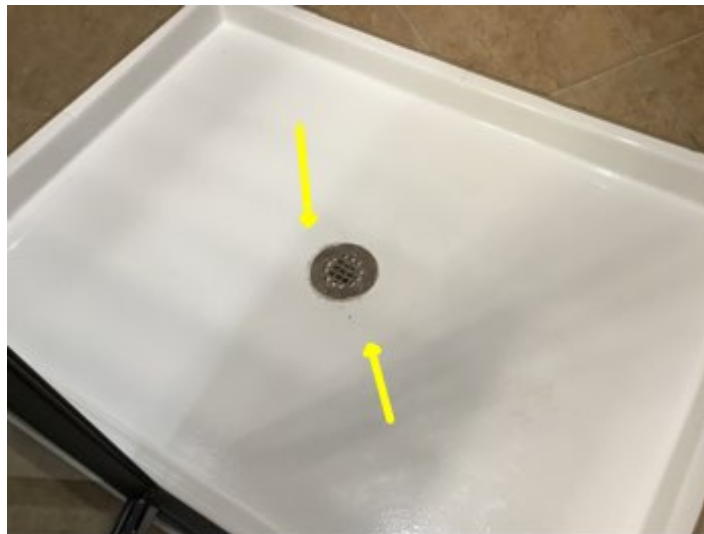
Cover for shower drain should be removable
