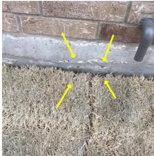
Exposed reinforcement
